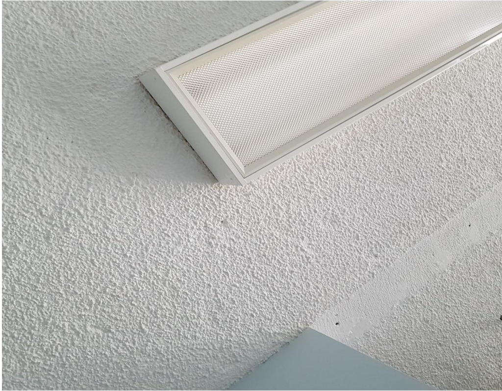
Figure 9: Plastered Ceiling (Potential Asbestos Concern)
