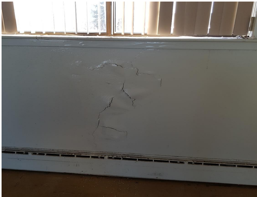
Figure 20: Water stain/damage on a wall near window (upstairs)
