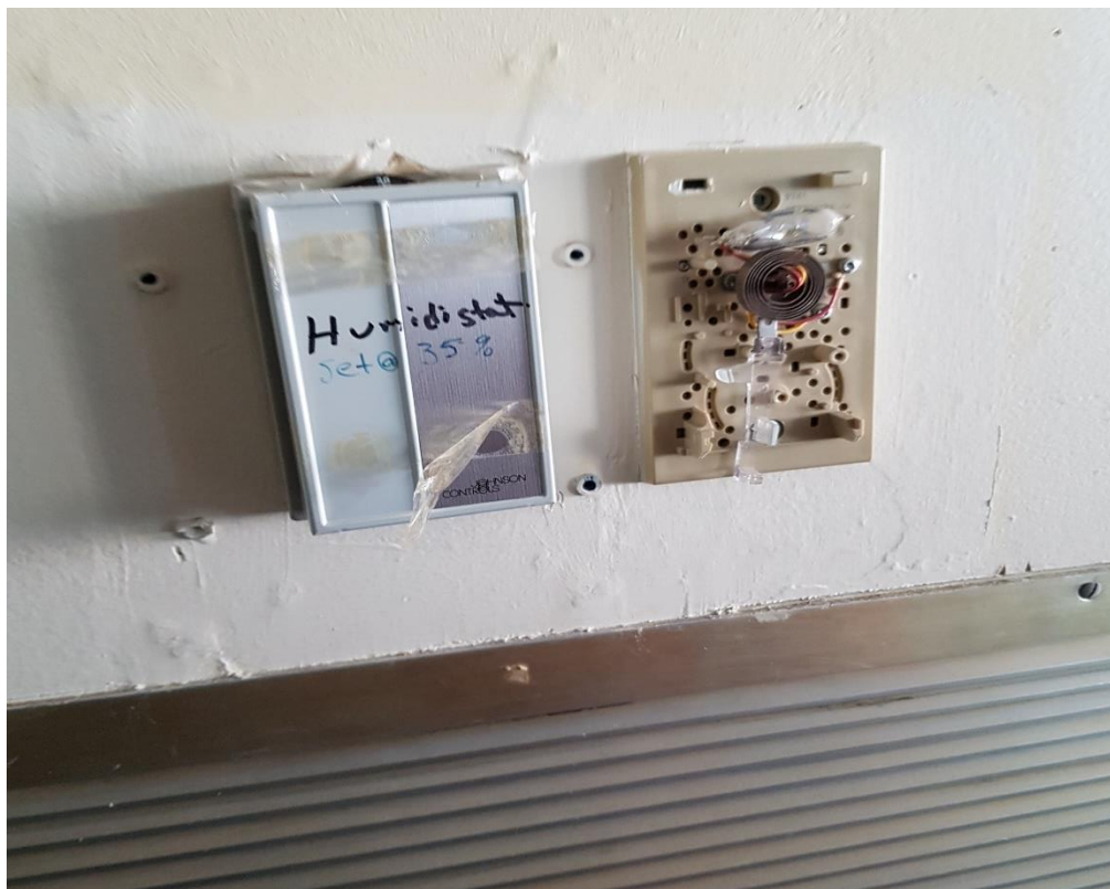
Figure 11: Switch containing Mercury
