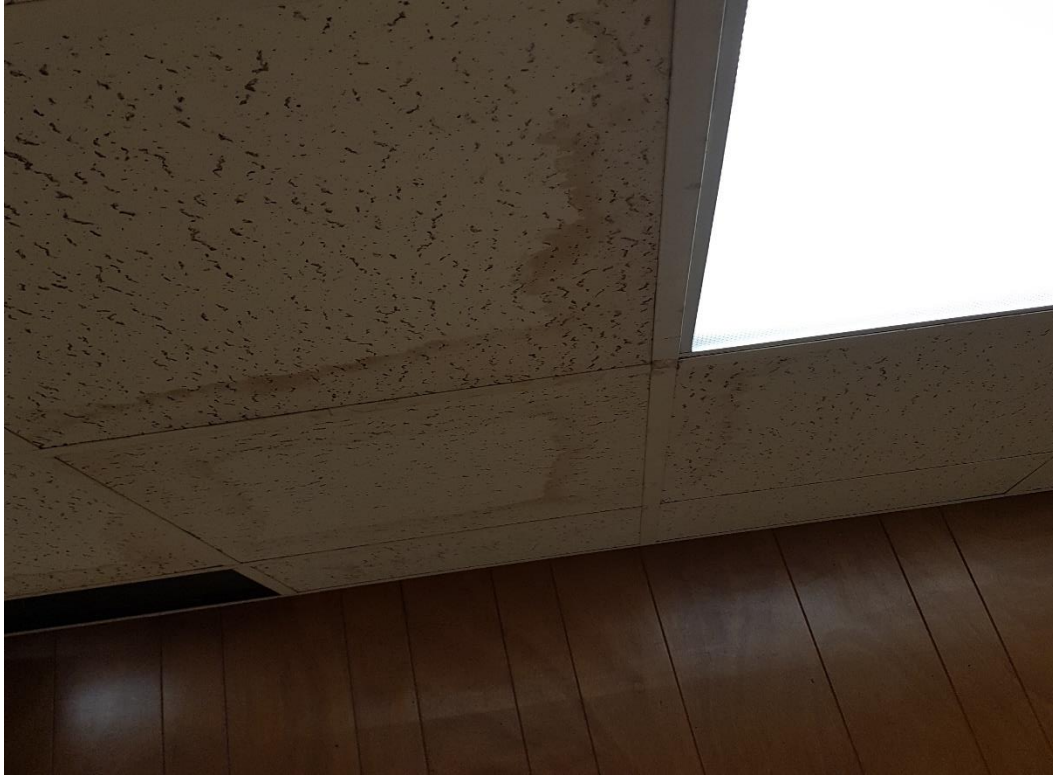
Figure 23: Water stained ceiling (basement)
