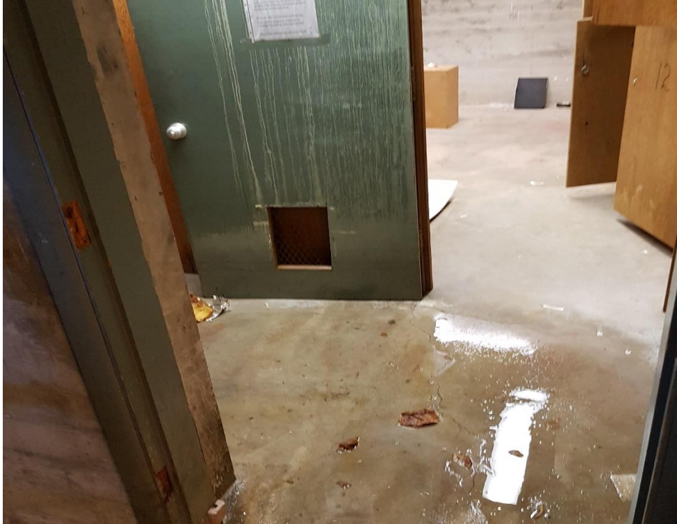
Figure 21: Pool of water from leaking pipe in basement area
