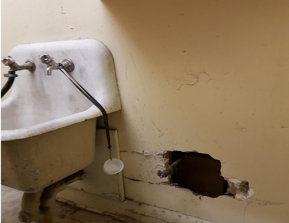
Figure 17: Hole in a wall (Janitor's Room)
