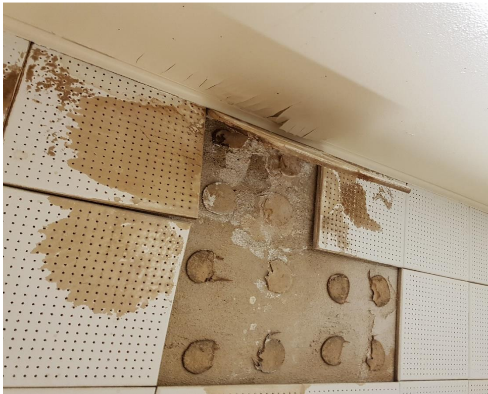
Figure 16: Water stained/ damaged ceiling
